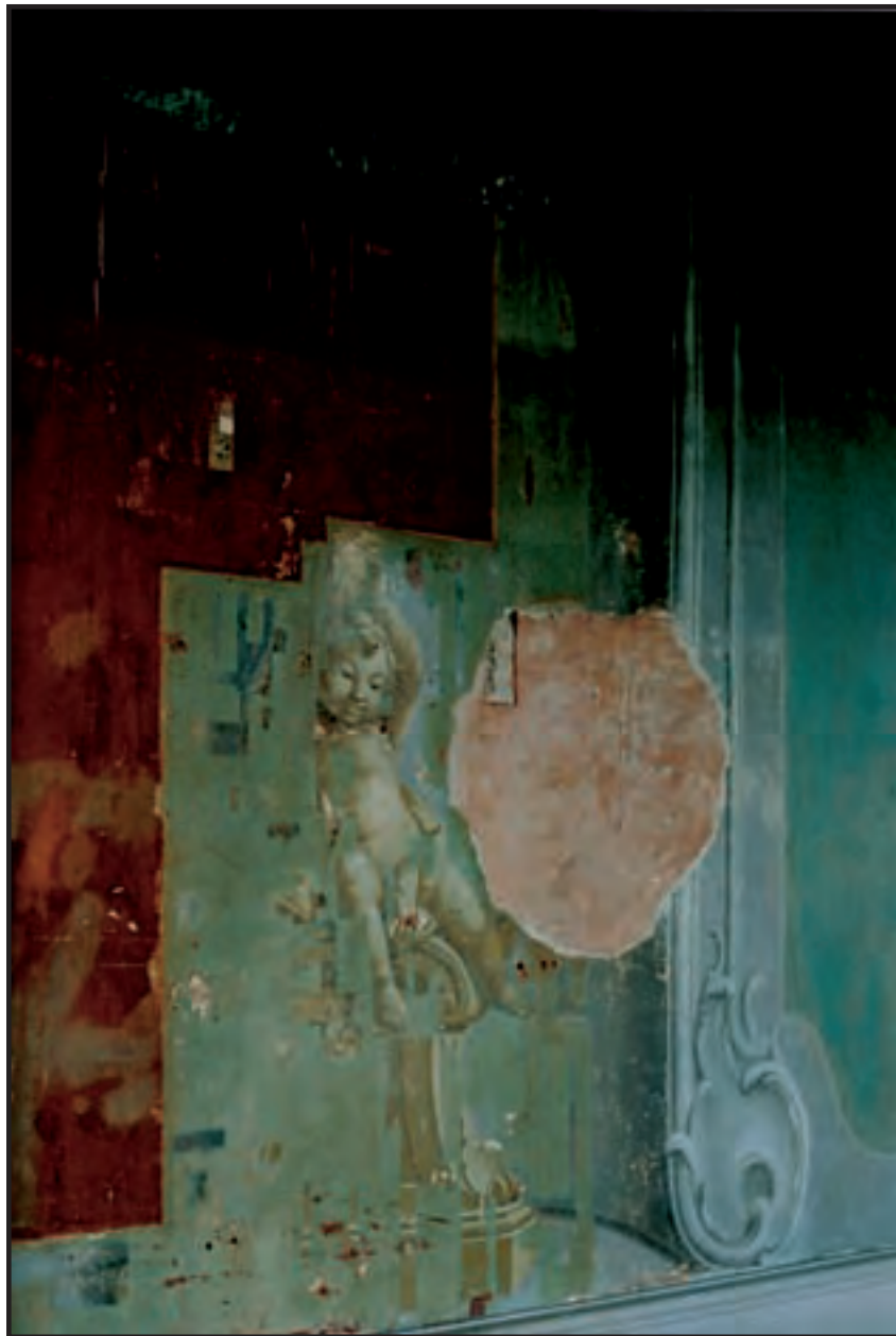
Layers of history – corridor in Rundale Castle 2001.
