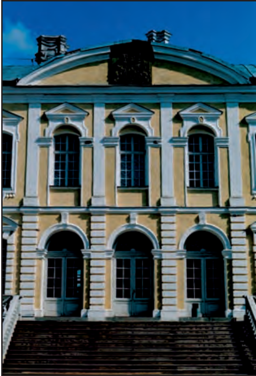
A national treasure is restored: Part of Rundale Castle under rehabilitation 1993.
